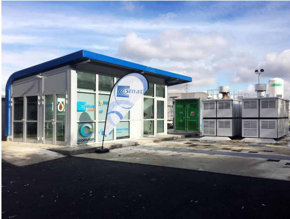
Figure 2. The two SOFC units of Convion installed on site.
