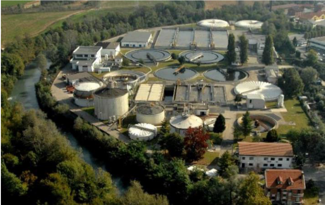
Figure 1-Collegno WWTP aerial view
