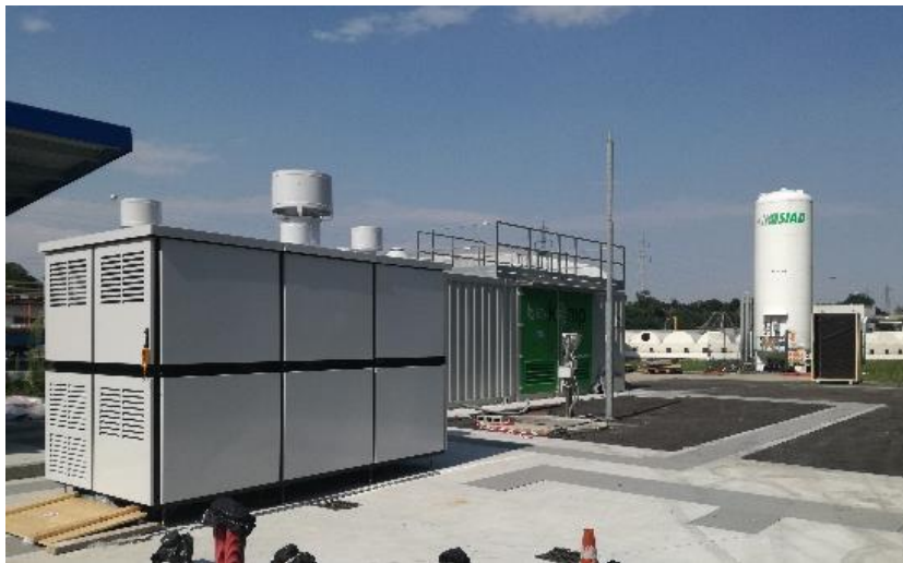
Figure 10. Shipment and installation of the first SOFC1 module.
