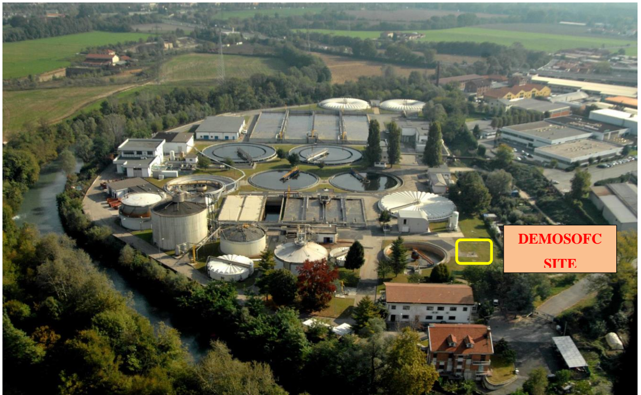
Figure 1. WWTP of SMAT Collegno (TO)
