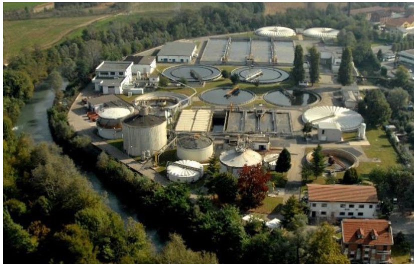
Figure 1. SMAT Collegno WWTP. Aerial view.
