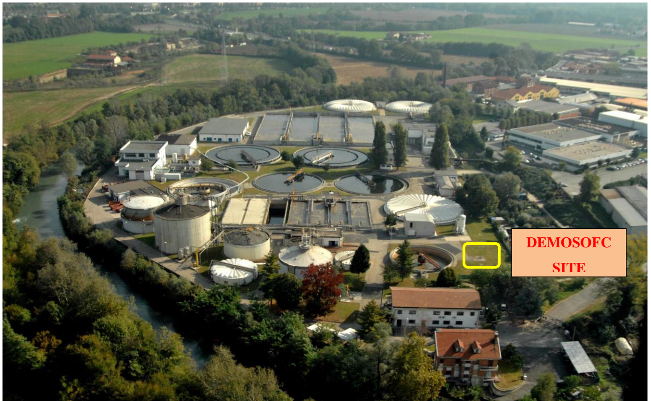
Figure 1. WWTP of SMAT Collegno (TO)
